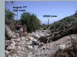
Marijilda Canyon showing high water from August 17, 2004 event. One quarter mile upstream, USGS slope-area estimated peak discharge of 6,800 cfs +/- 20%. Photo by USGS.
