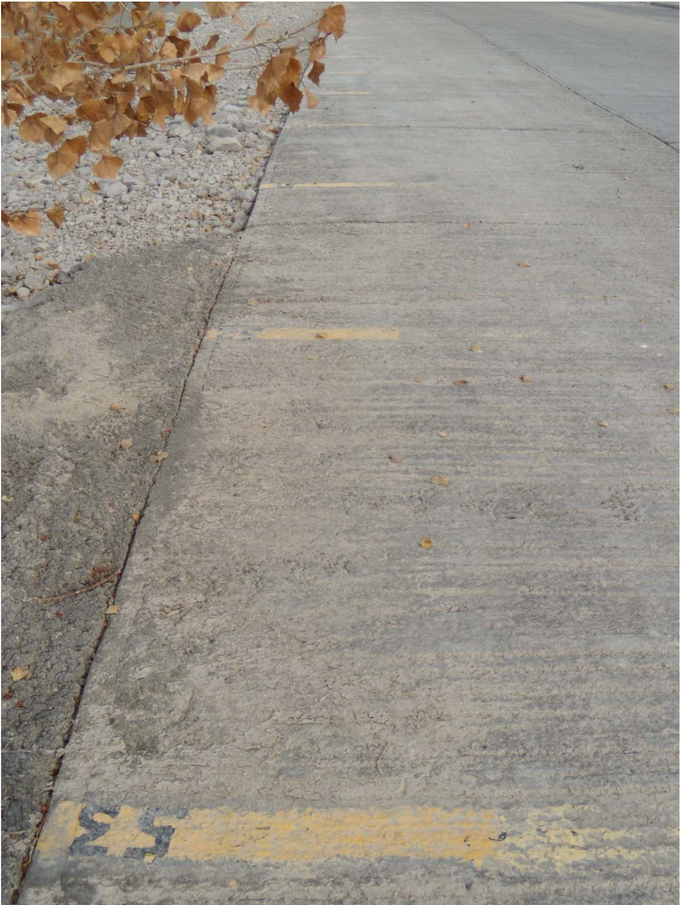
Photo 12: Painted inclined staff gage along edge of Millsite Reservoir boat ramp. EWCD website reported 31.58 feet; therefore, the reservoir level was ~21.5 feet below this point near top of boat ramp. Tim Bardsley, November 12, 2009
