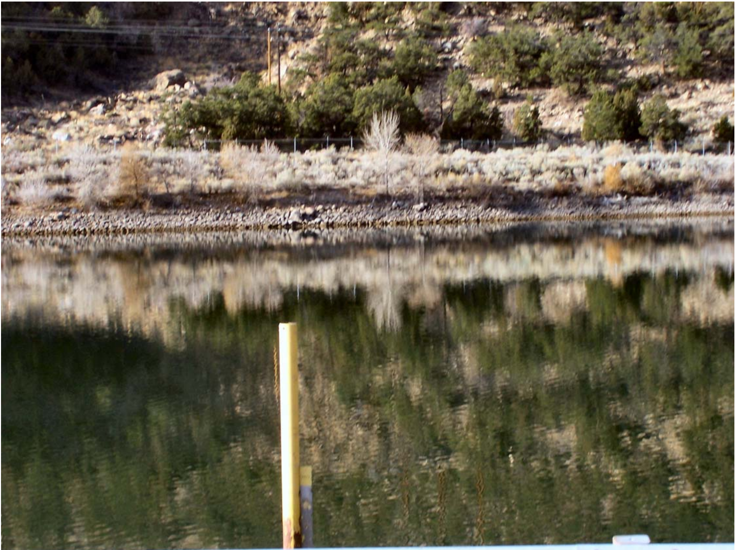
Photo 1: Holding Pond for Power Plant Diversions.
