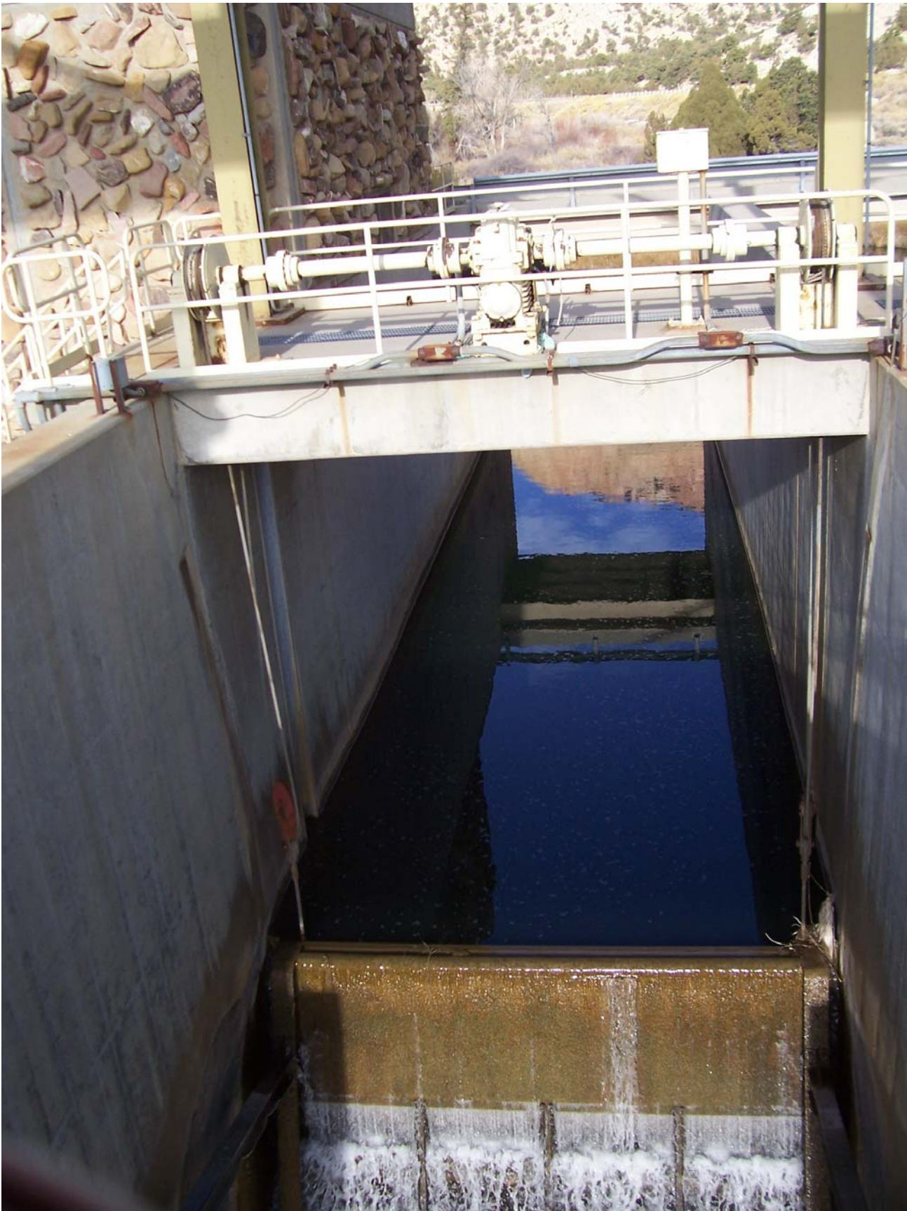
Photo 4: Control structure for Power Plant diversions upstream of gage. (N 39° 23.455', W 111° 05.550', elevation: ~6509 ft.) Inside of building not visited.
