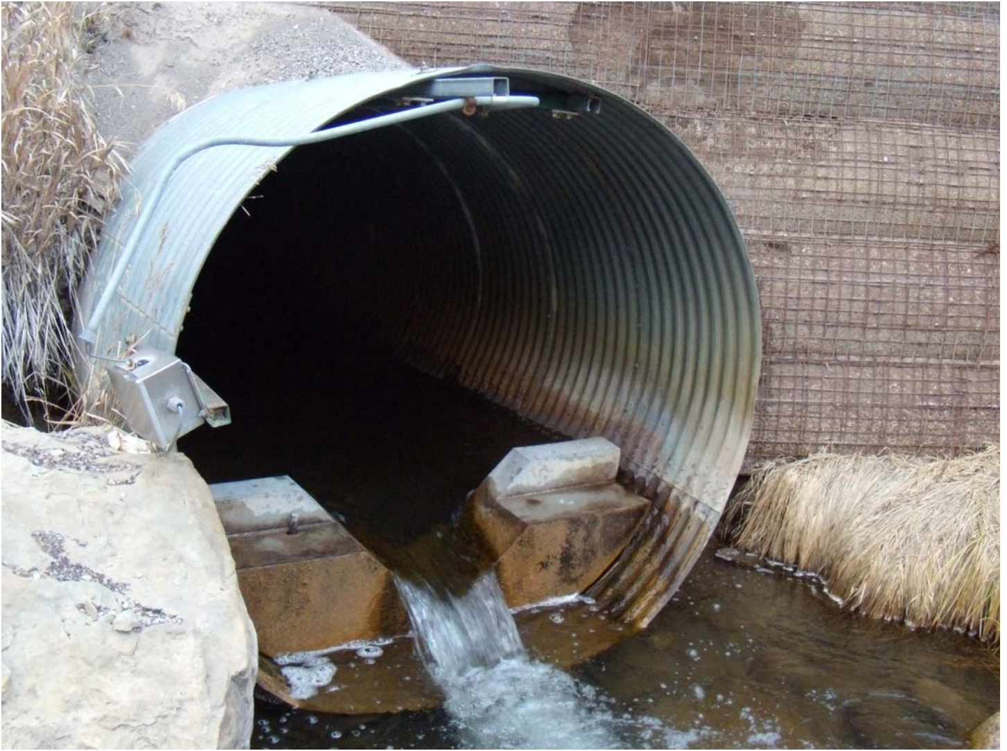
Photo 33: Boulger Creek, tributary to Electric Lake. Gage is in culvert under State Route 264. Tim Bardsley, November 12, 2009
