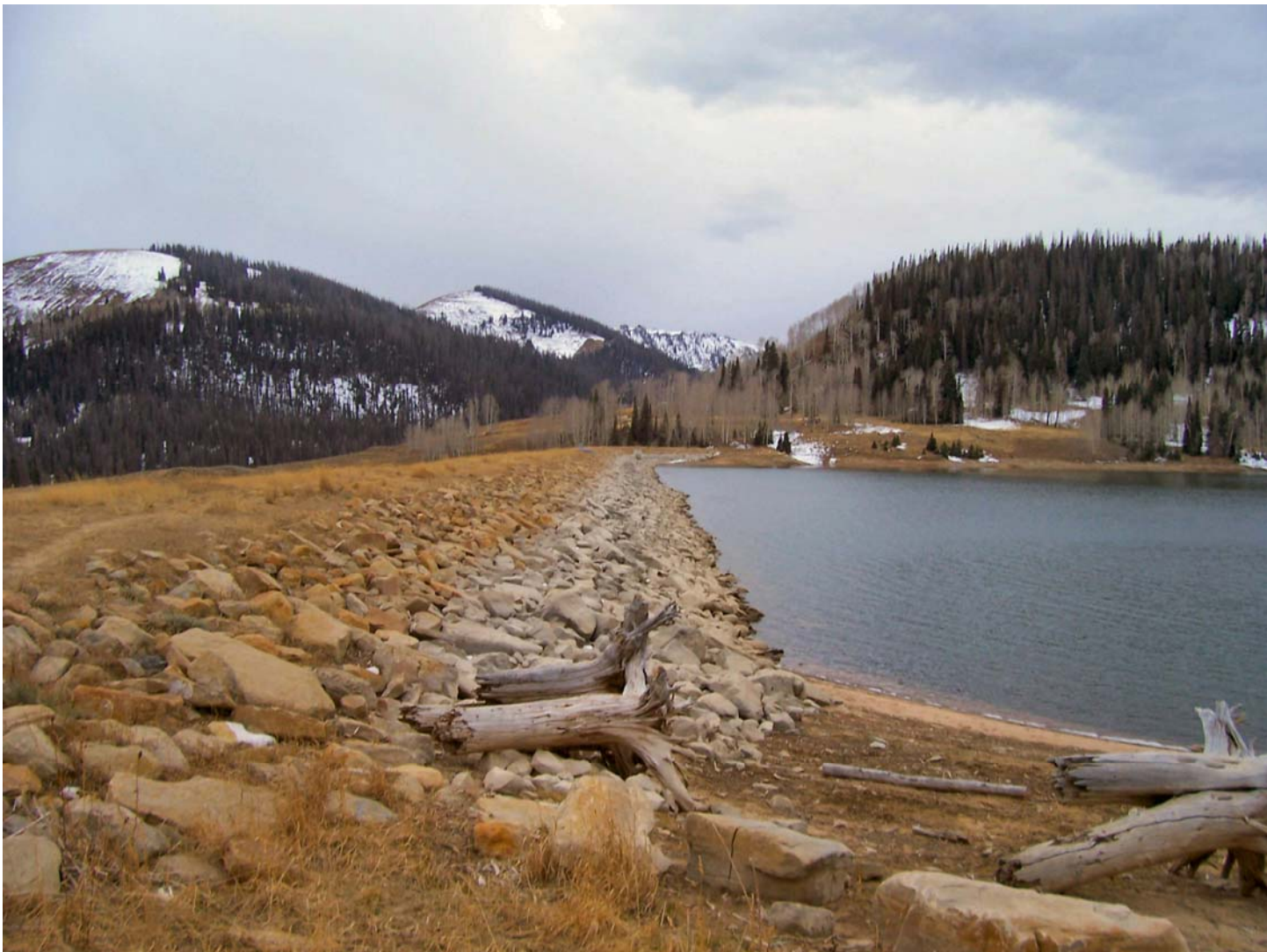
Photo 31: Huntington Reservoir and dam.
