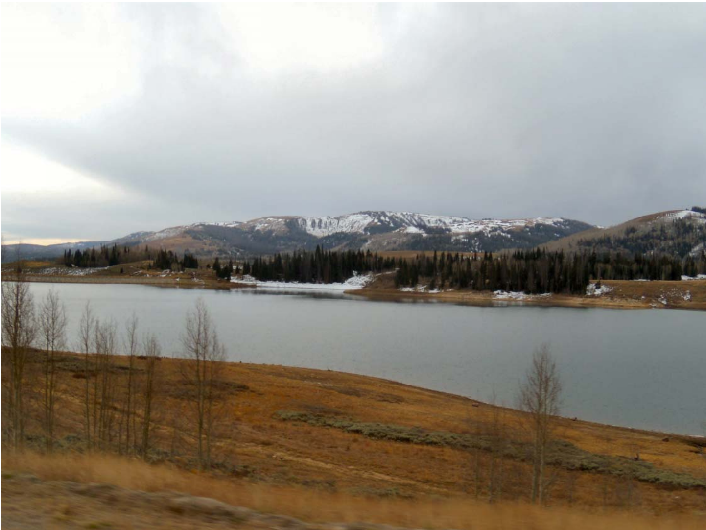
Photo 28: Cleveland Reservoir looking towards dam
