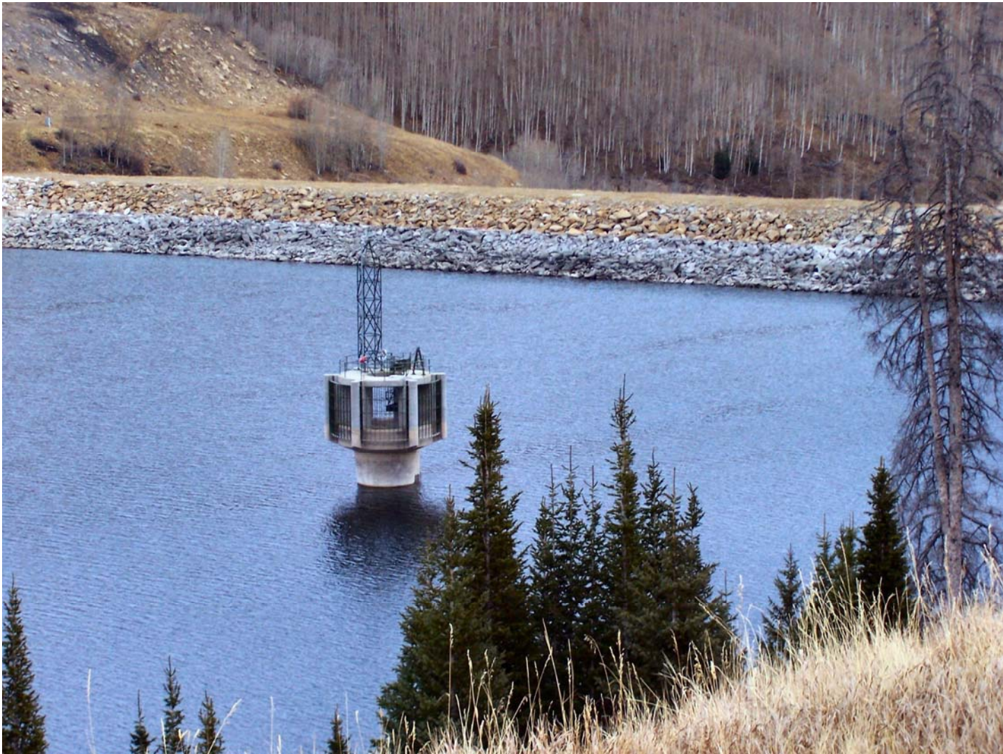
Photo 29: Electric Lake and dam.
