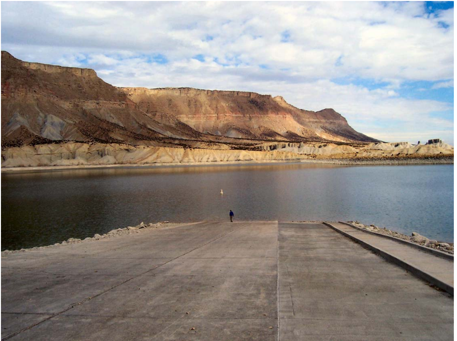
Photo 9: Millsite Reservoir, painted inclined staff gage along edge of this boat ramp.
