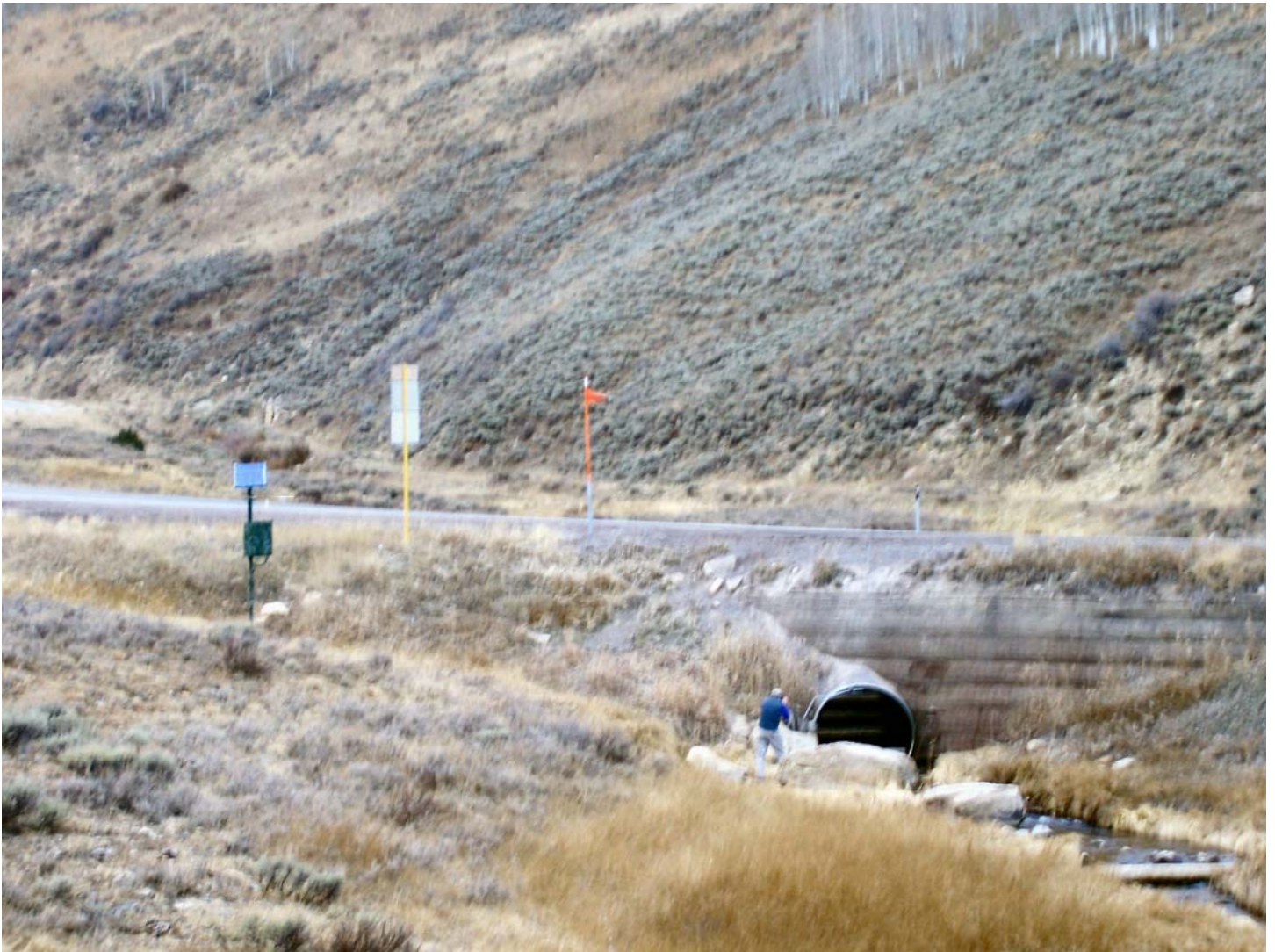
Photo 32: Boulger Creek, tributary to Electric Lake. Gage is in culvert under State Route 264. William Reed, November 12, 2009
