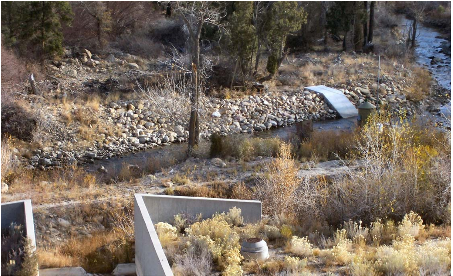
Photo 2: Spillway for holding pond at bottom left, old USGS gage right of center, new gage right of USGS gage. Flow is from left to right.
