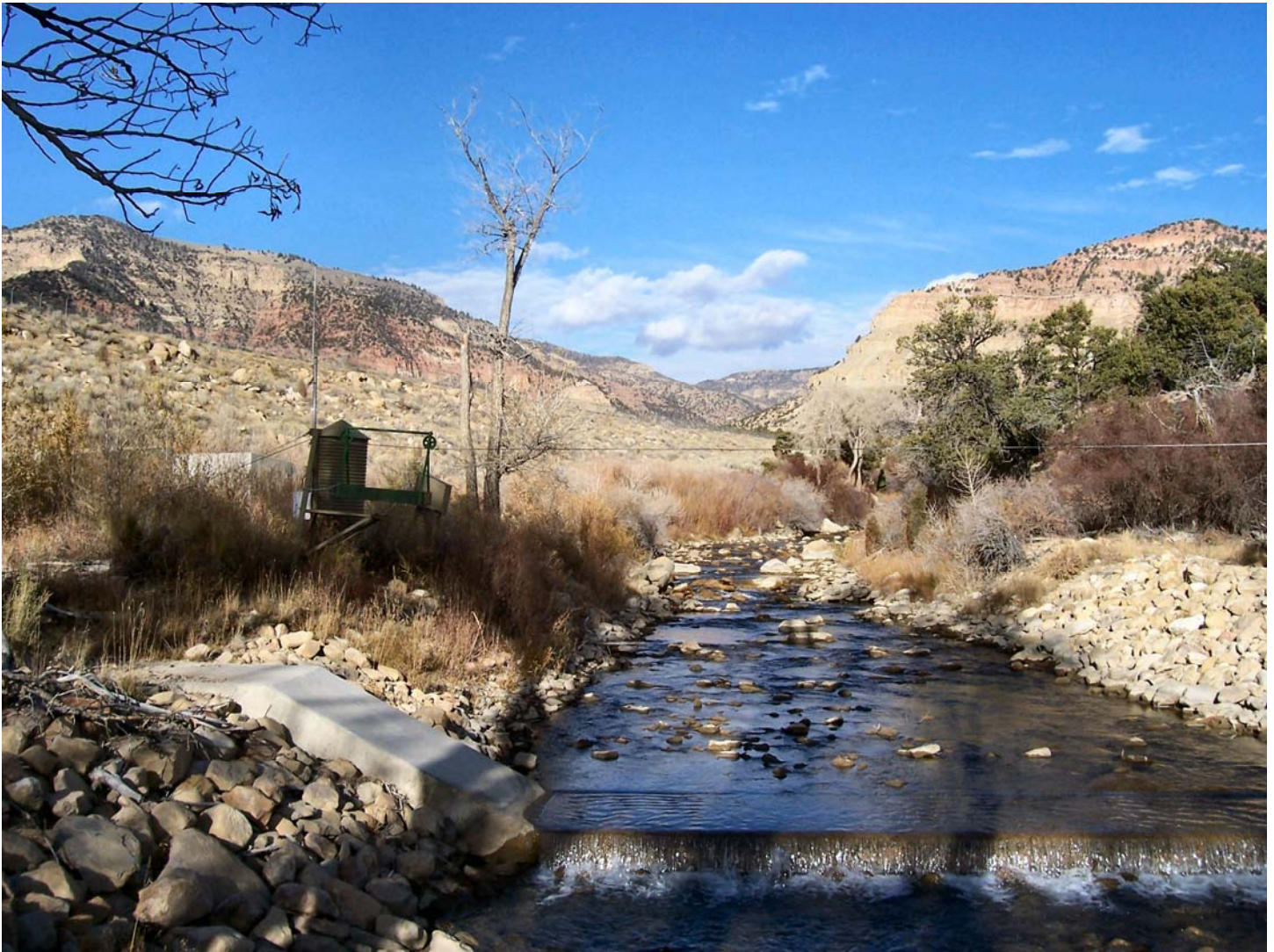
Photo 6: Huntington Creek gage, looking upstream, showing control for gage in foreground. William Reed, November 12, 2009
