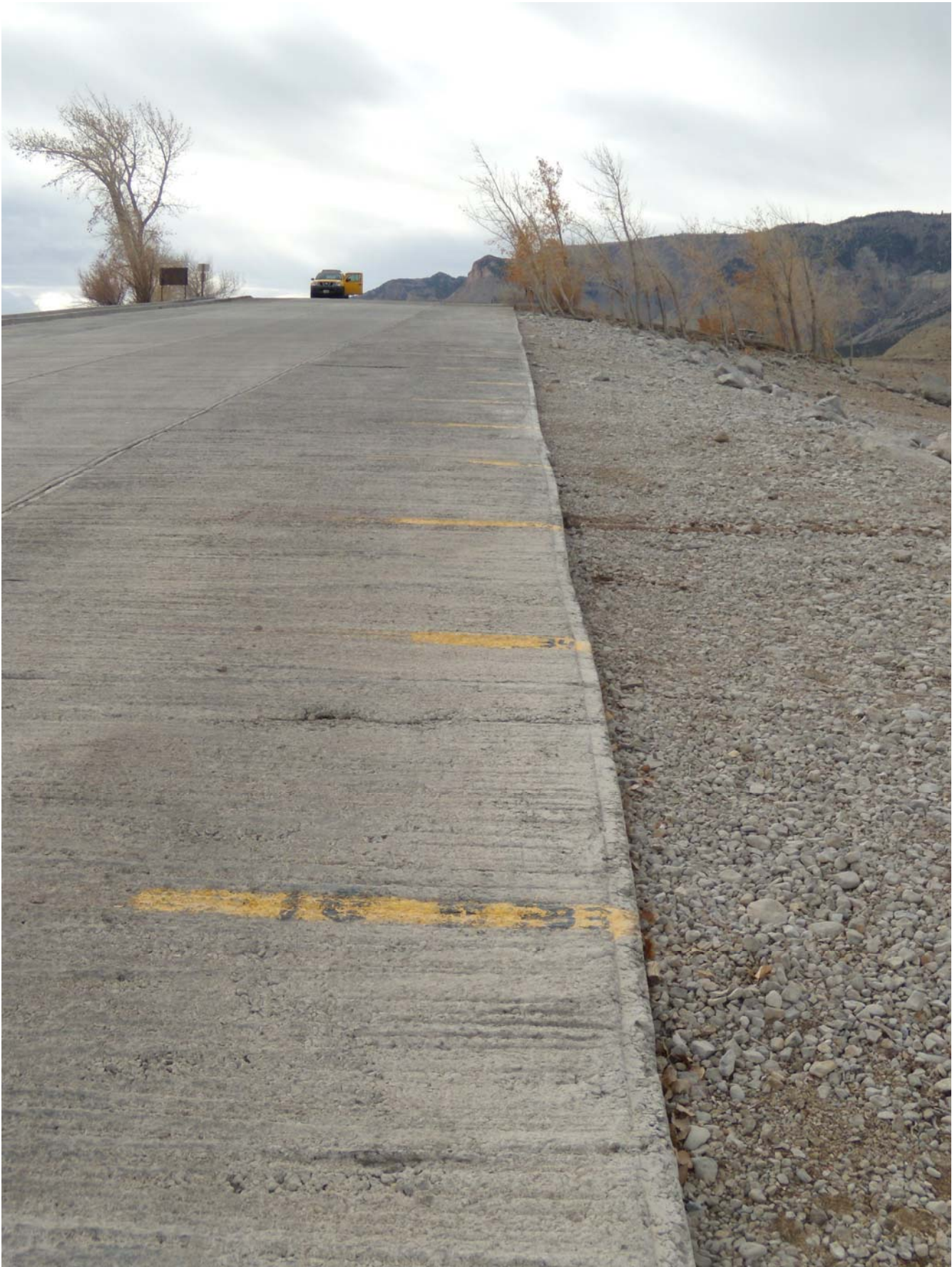
Photo 11: Painted inclined staff gage along edge of Millsite Reservoir boat ramp.
