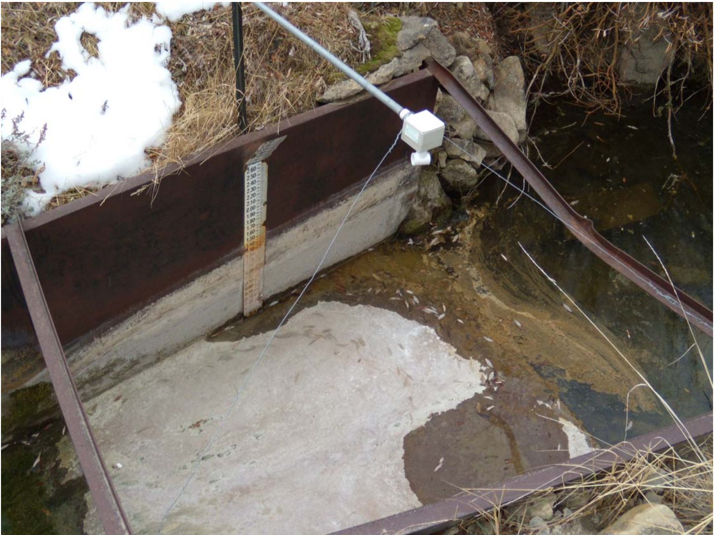
Photo 25: Rolfson Reservoir Dam outflow gage.
