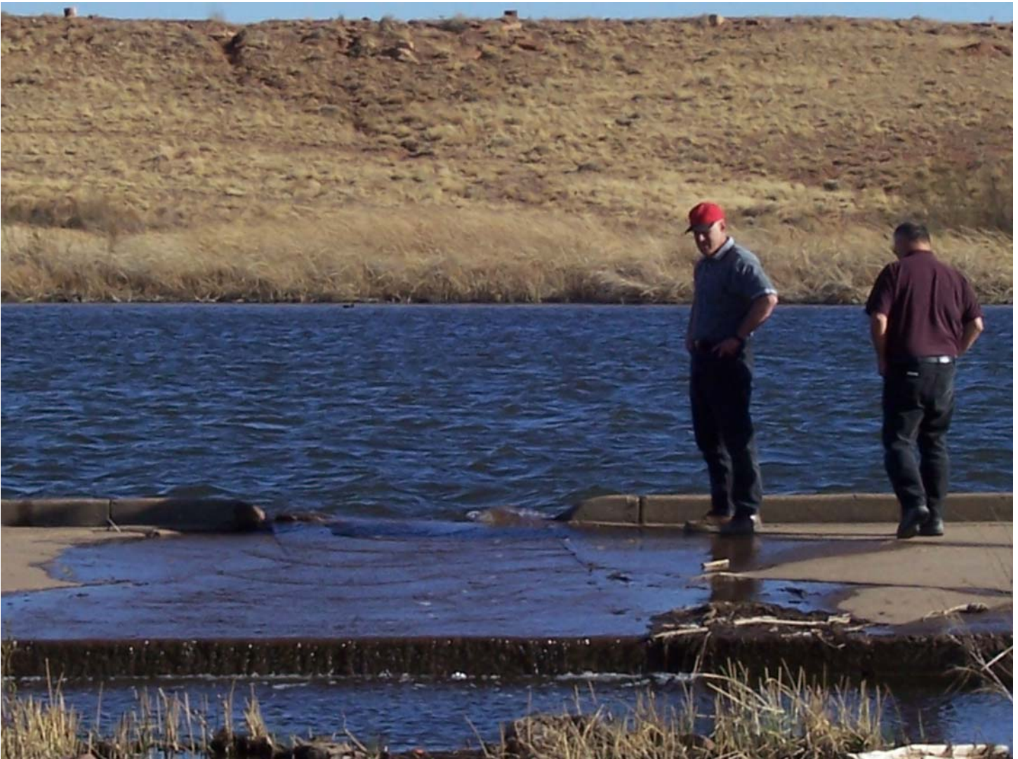
Outlet for Clear Creek Reservoir, a.k.a. McHood Lake, looking towards lake. Flow was 0.5 to 1.0 cfs. 4/11/2006.
