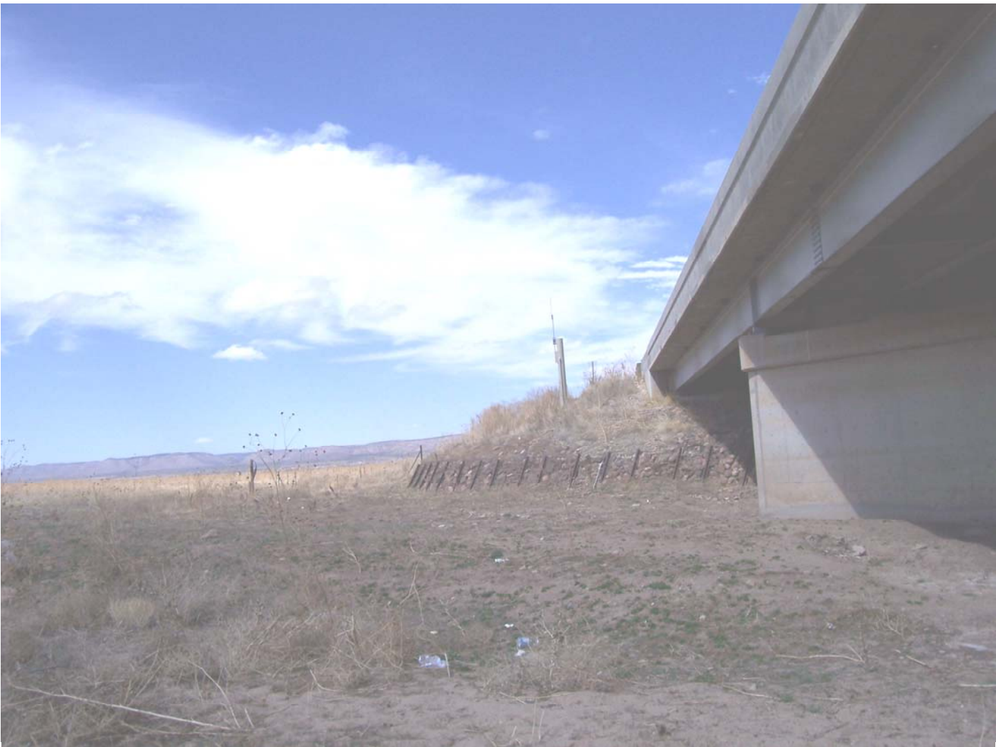
Big Chino Wash looking toward gage on left bank and upstream of bridge. 4/10/2006.
