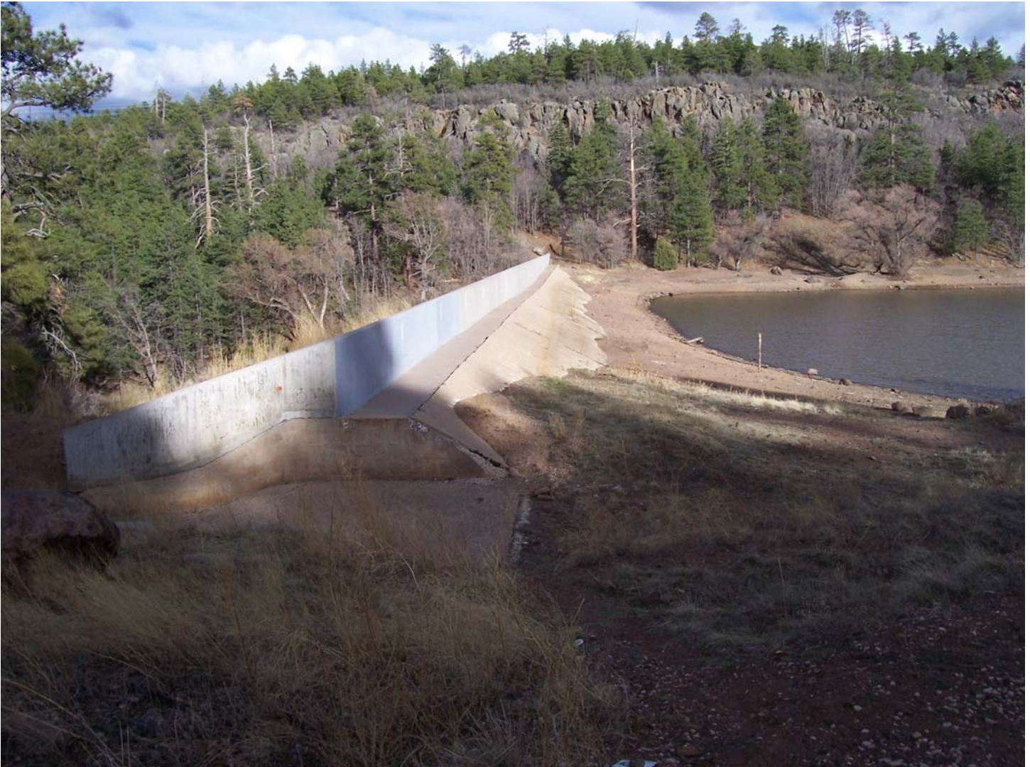
City Dam looking at spillway and existing ponding behind dam. ALERT gage is located on far bank (right bank) and has no Hand Book 5 ID. 4/10/2006.
